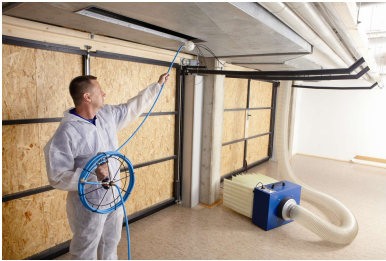
Fig. 16: Cleaning ductwork with a roller guide ball and compressed air whip, dirt extracted with dust collector
