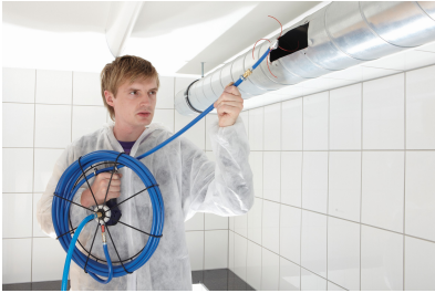
Fig. 5: Application example: Cleaning ventilation ducts
